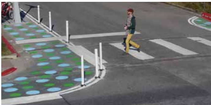
Piloting a curb extension using paint and plastic bollards in Austin, Texas. Image: Streetsblog
